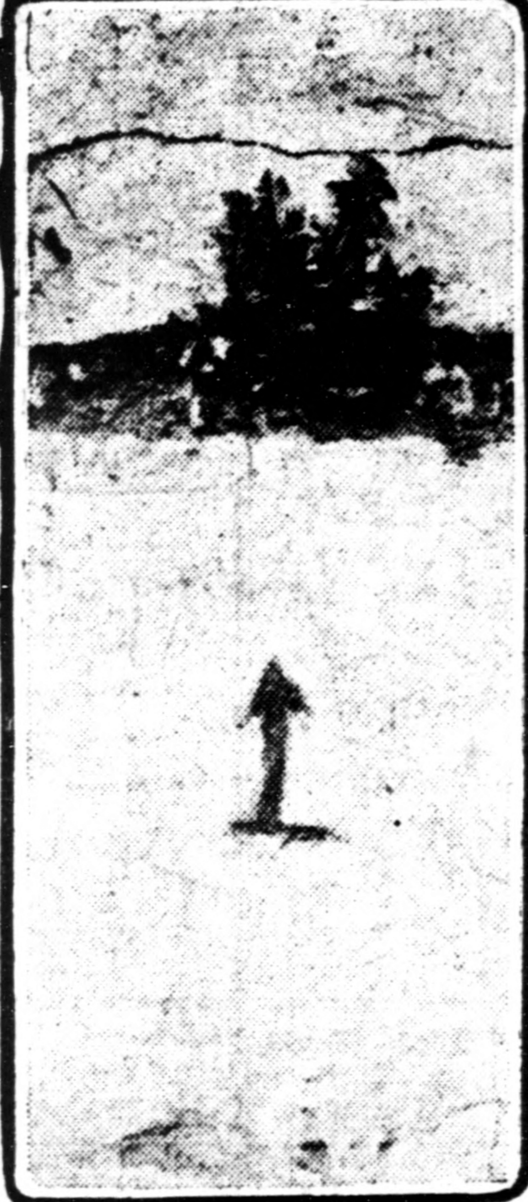
Engineer's Mark on Sea Wall, Indicating Whereabouts of Landmark.
